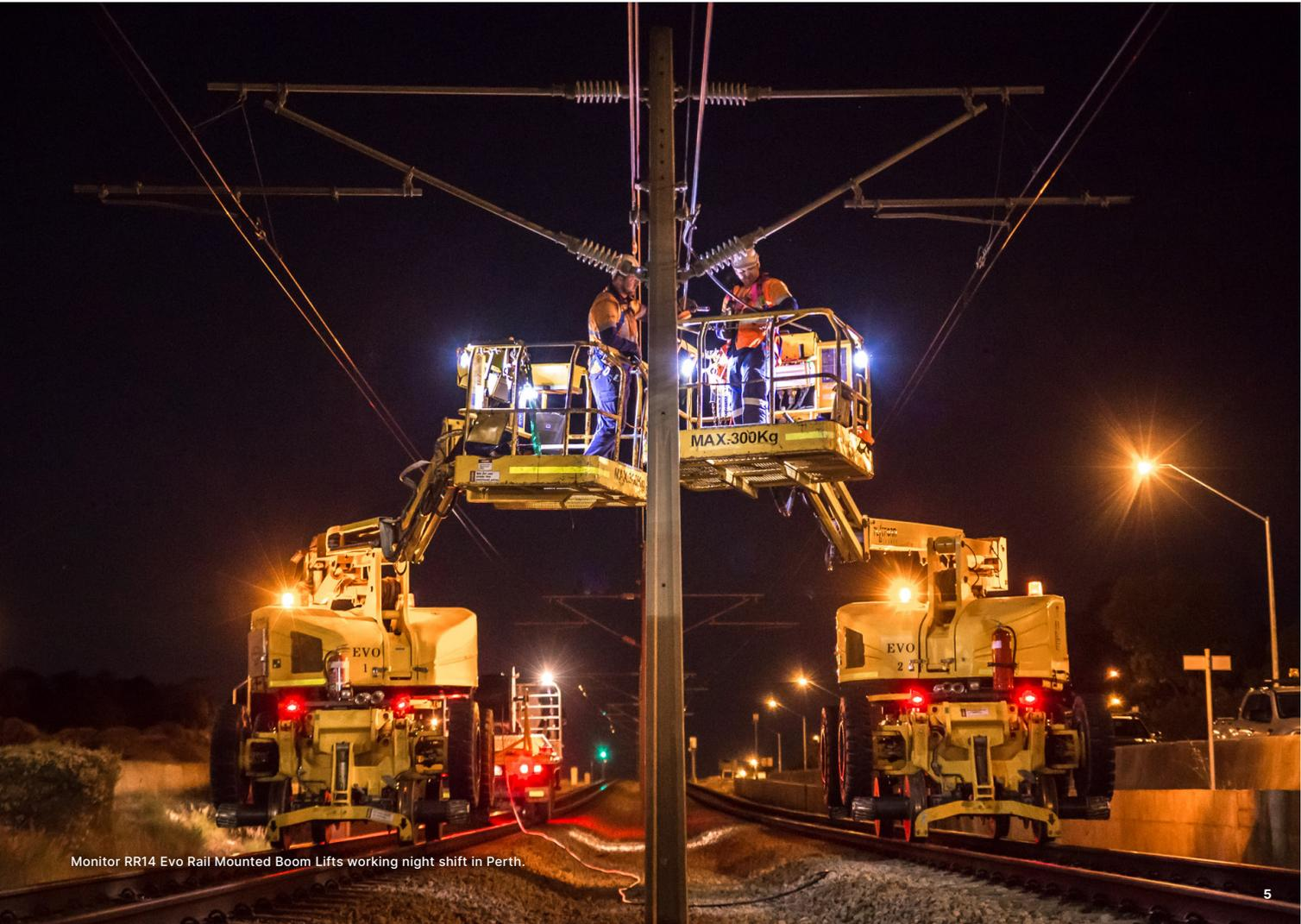
Monitor RR14 Evo Rail Mounted Boom Lifts working night shift in Perth.
